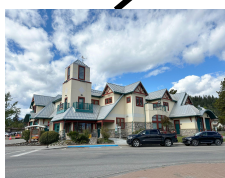
Emergency Services Building 518 Geike Street
