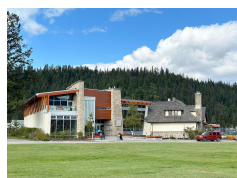
Library and Cultural Centre 500 Robson Street
