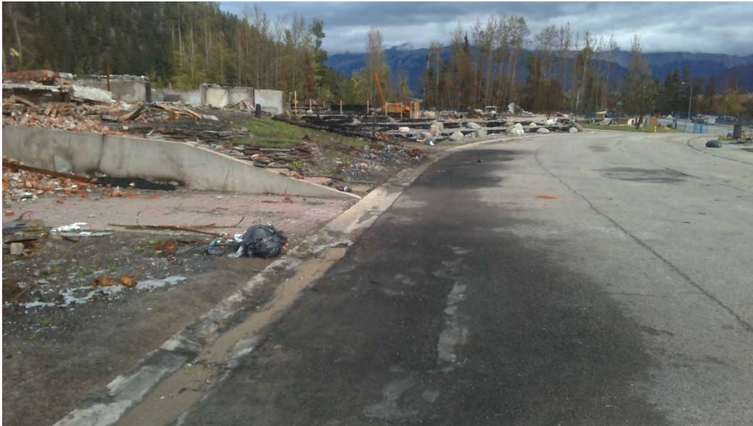
Pictured above: Damaged curb and gutter on Cabin Creek Drive
