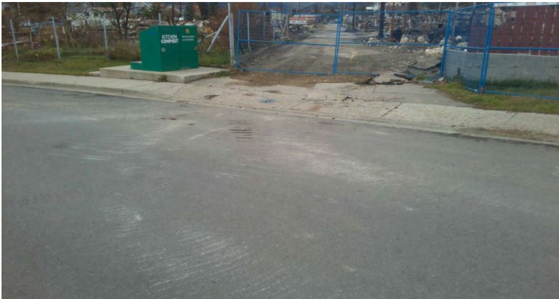
Pictured above: Damage to laneway crossing by tracked equipment
