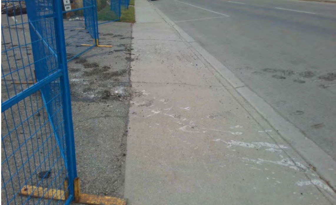
Pictured above: Commercial entrance damaged by tracked equipment
