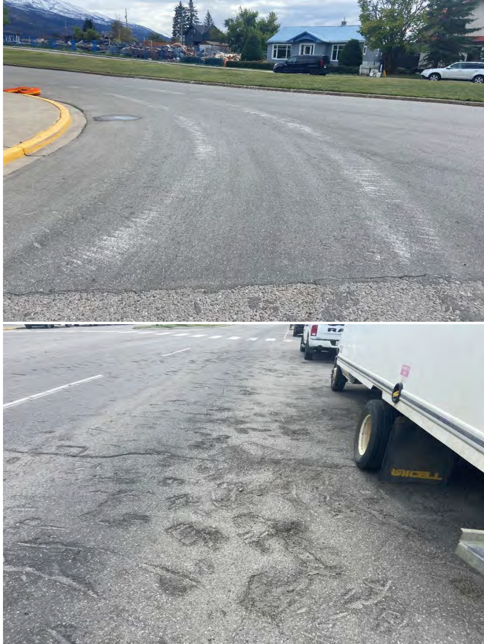
Pictured above: Typical damage to roadways including burned asphalt, gouged asphalt, and track damage from heavy equipment.
