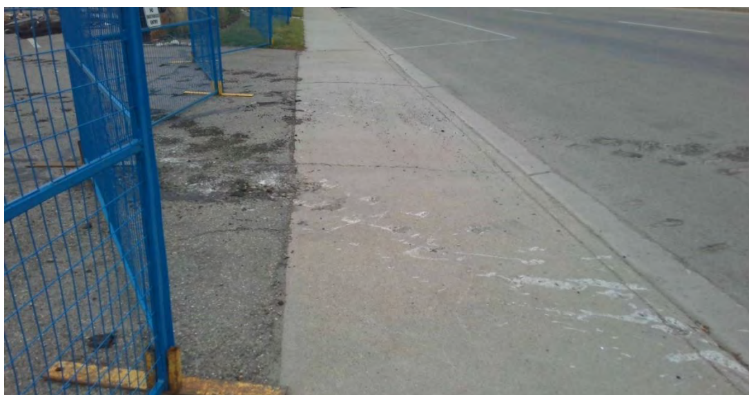
Pictured above: Typical damage to sidewalk caused by heavy equipment
