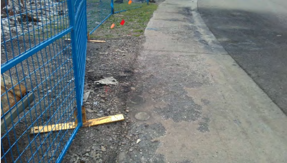
Pictured above: Sidewalk damage caused by intense heat of fire
